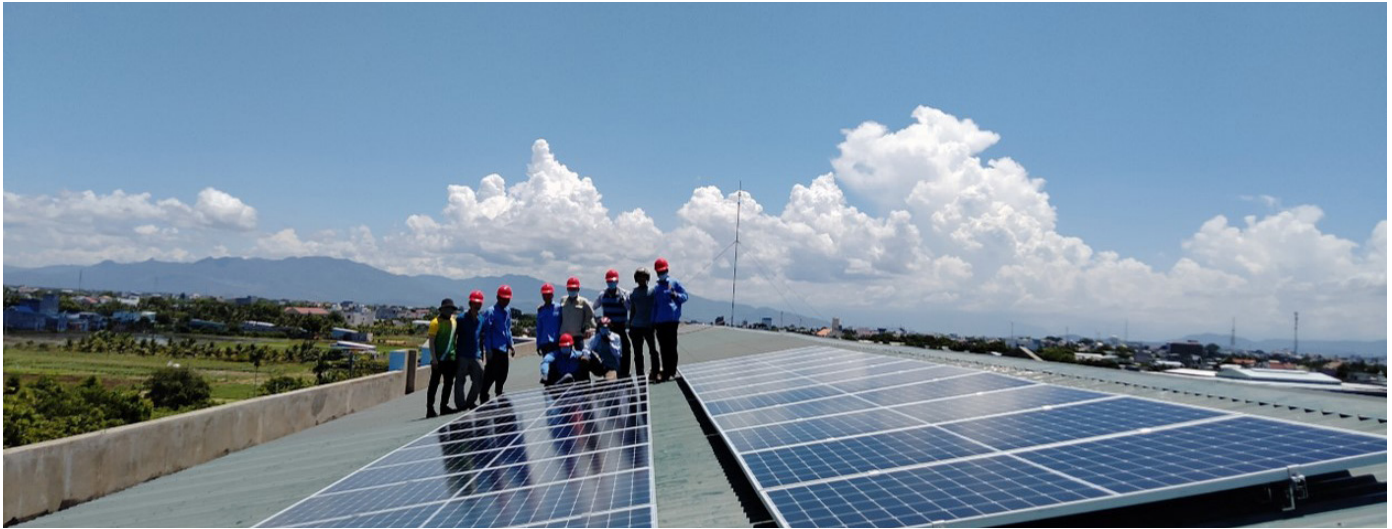
Teachers of Ninh Thuan Vocational College Install the 10 kwp grid-connected roof top solar system on the roof of a practical training workshop.
